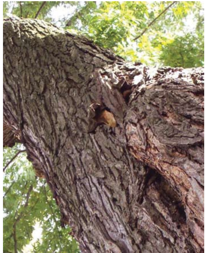
Closeup of a long exposed leader of a silver maple ( Acer saccharinum ), showing a large spiraling crack with an associated fungal fruiting body (prob. Polyporus squamosus ). This damage was likely caused by large rotational stress. (Photo by Jerry Bond)
